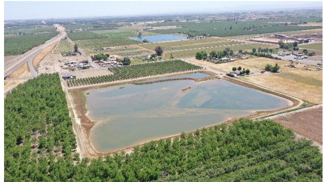
Laguna Irrigation District's 30-acre Casa Loma Pond in the foreground and 20-acre Vaz Pond in the distance. Casa Loma recently underwent improvements ahead of this wet year to increase the rate water is recharged into the aquifer. Laguna ID is a member of the North Fork Kings GSA.
