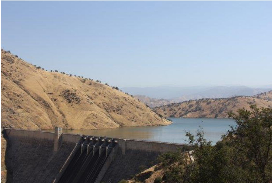
Pine Flat Lake and Dam peak storage June 2024
